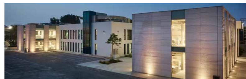
BESIX 3D printed the largest 3D printed concrete façade in the world for the new Dubai headquarters of BESIX in 2020. Results: use less concrete and carbon footprint reduction with more complex shape opportunities.
