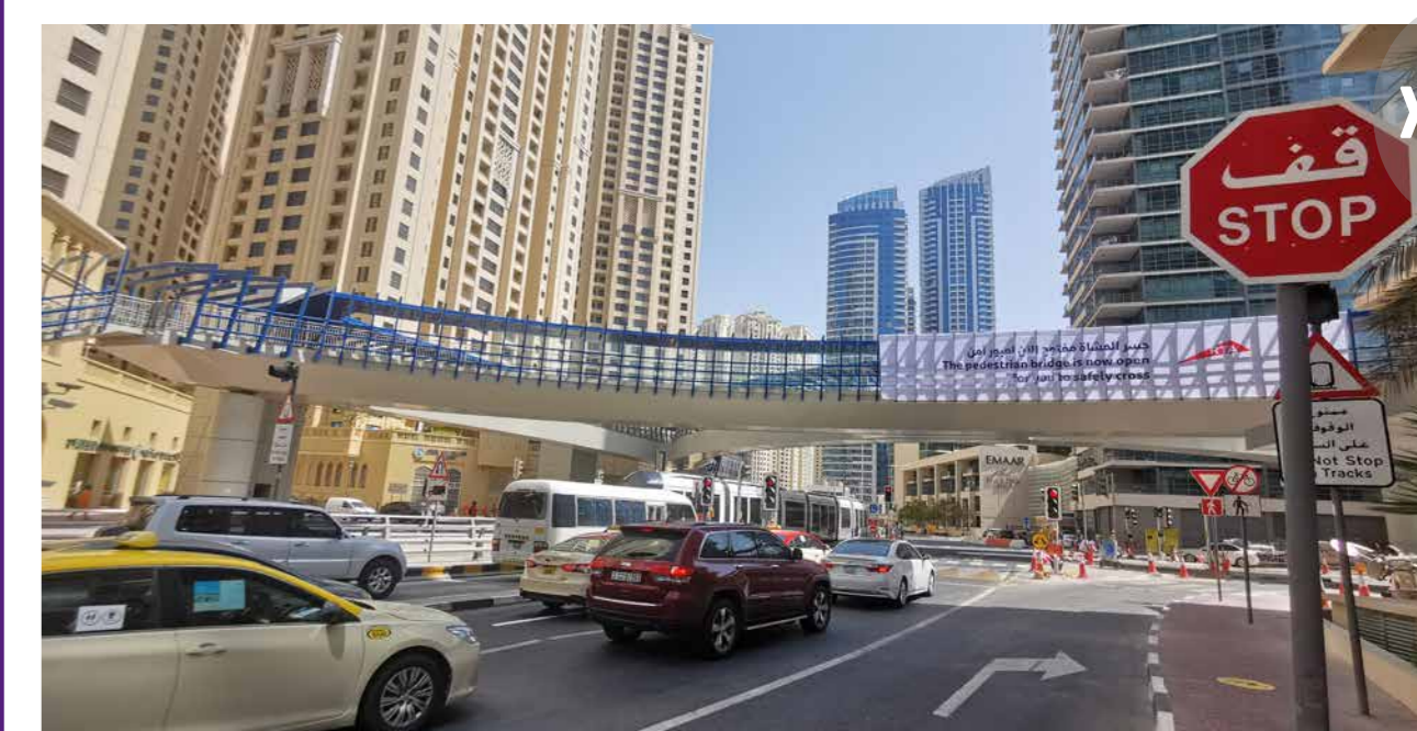
Dubai pedestrian bridge (UAE) – A four-way footbridge (75 m length) that allows +8,000 pedestrians to safely cross one of the busiest junctions in Dubai. This project is to be part of the Dubai Roads and Transport Authority’s plans to rank among the world’s safest cities in traffic safety by 2021.
